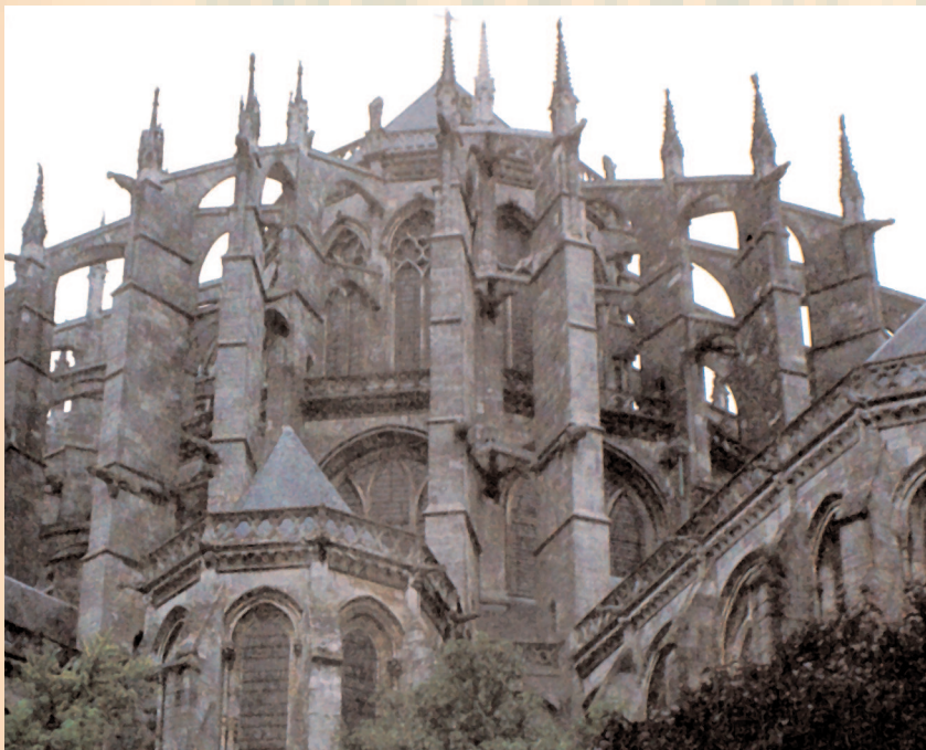
Fig 37. Le Mans Cathedral, 11th Century France. Also known as the cathedral of St Julien. The edifice consists of Gothic architecture superimposed over the original Romanesque structure, which was gutted by fire on two different occasions, the second being in 1134 contemporaneously with the destruction of Chartres Cathedral.
